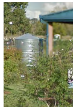
Existing Cistern and Irrigation
