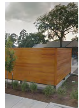
Dumpster with Wood Enclosure
